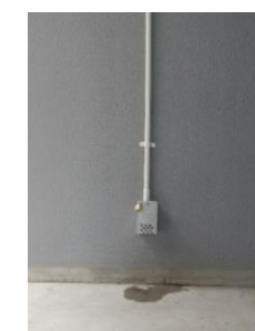
Installation of flood sensors
