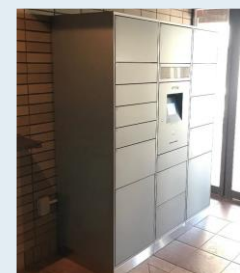
Installation of additional parcel boxes
