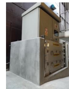
Installation of water stop
